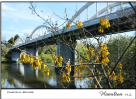
Fairfield Bridge C.PC.WAI.13
