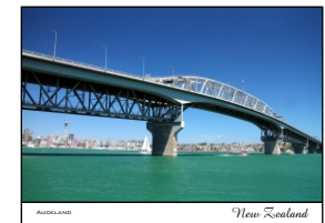
Harbour Bridge C.PC.AKL.68
