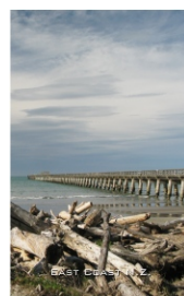
Tologa Bay Wharf MG.59.EC.03
