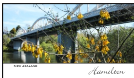
Fairfield Bridge MG.95.WAI.13
